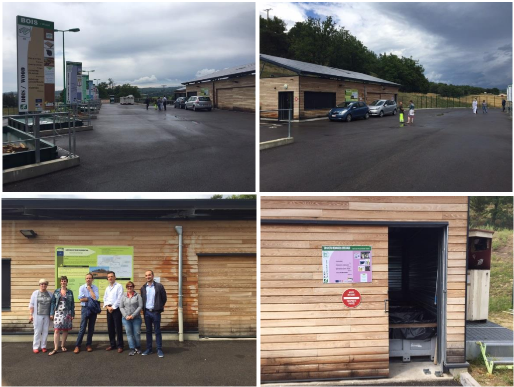
Figure 2. Ecopoint of the LIFE CCHP.
